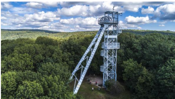
Ratzinger observation tower is a retrofitted former mining elevator tower
