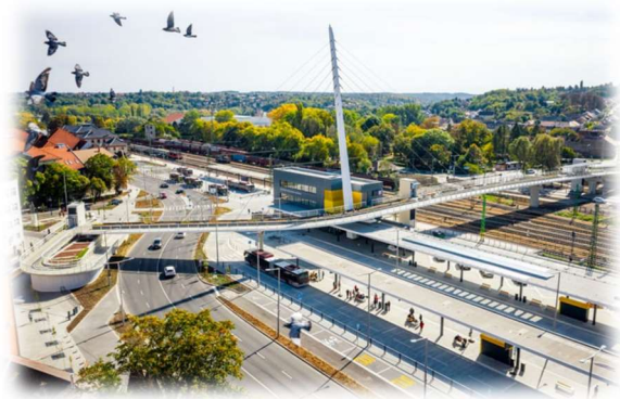
The new Intermodal Hub finished in 2020 - just 350m from the Main square
